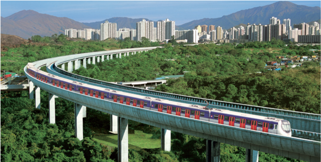
West Rail linking Nam Cheong and Tuen Mun, seen running on viaduct
