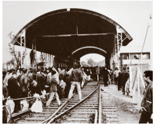
Passengers crossing the old Lo Wu bridge to the Mainland
